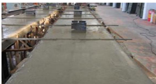
Fig. 2. Image of the beam after concreting.
