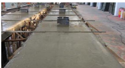
Fig. 2. Image of the beam after concreting.
