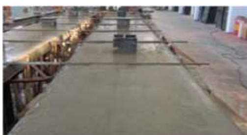
Fig. 2. Image of the beam after concreting.
