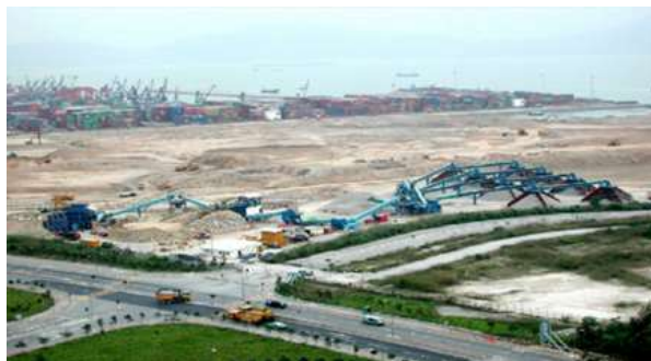
Fig. 1. A picture of a concrete recycling center in Hong Kong.
