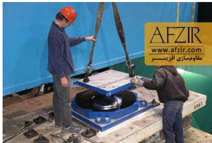
Fig. 4. Installation of pendulum separators.
