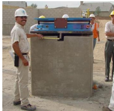
Fig. 3. Friction pendulum seismic isolator system (FPS).
