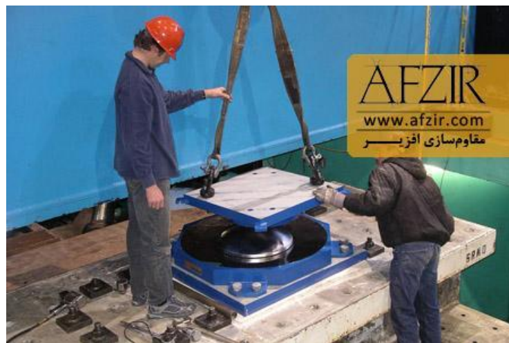
Fig. 4. Installation of pendulum separators.
