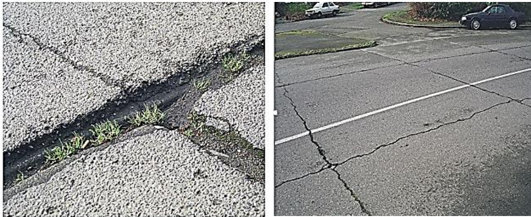
Fig. 8. Reflective cracking [61].
