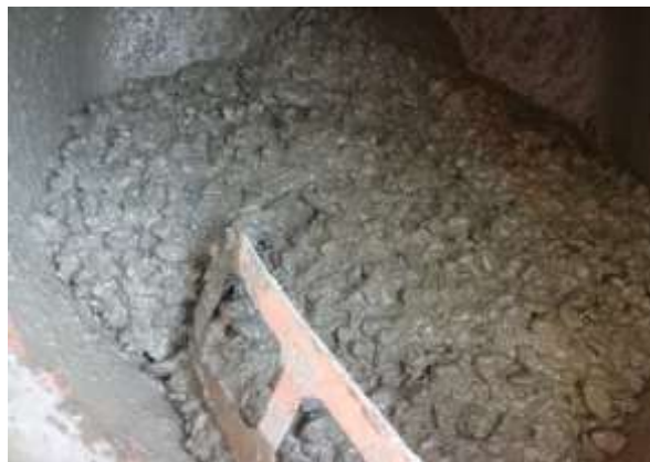
Fig. 6. Fresh concrete after compaction in molds.
